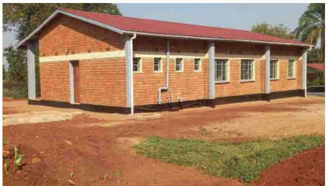
Newly built VSU in Mulanje
